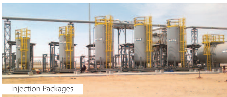
Antifoam, Antiscale, Ferrous Sulphate and Sodium Sulphite Dosing Package
