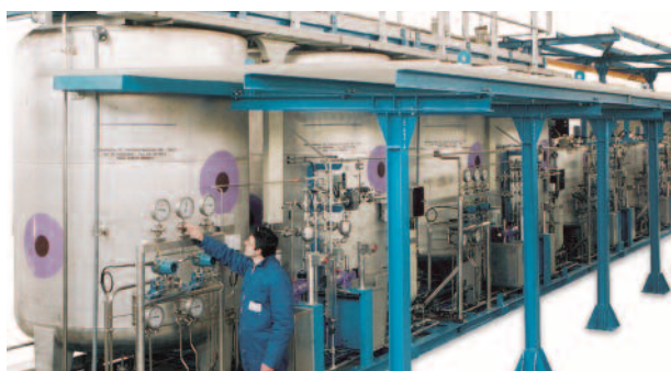
Antifoam, Antiscale, Ferrous Sulphate and Sodium Sulphite Dosing Package
